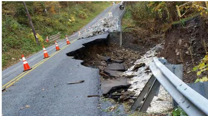
Purdue Mountain Road in Benner Township experienced significant road damage due to the October 20 storm, which FEMA subsequently dedicated \$1.2 million for the repairs.
