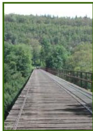
Viaduct bridge along Snow Shoe Rail Trail
